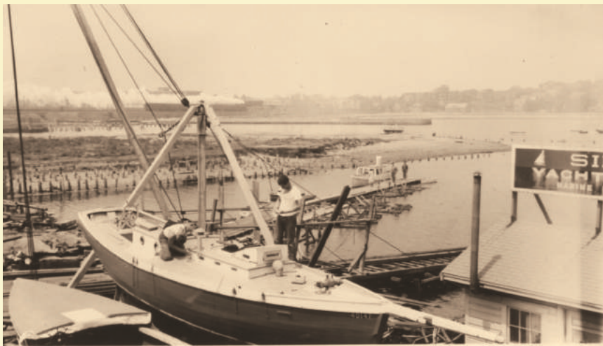
"stepping the masts the old fashioned way" - Fuller kneeling
