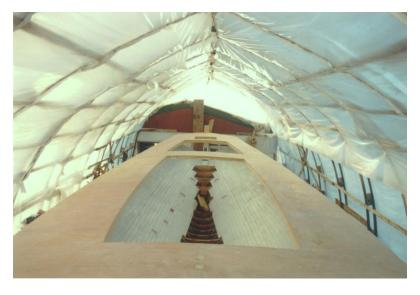
leak no matter how careful I was, so we are satisfied with our leak-free painted deck. I only wish that I had doubled up on the fibreglass on the foredeck and cockpit where heavy things with sharp edges seem to get dropped regularly.
