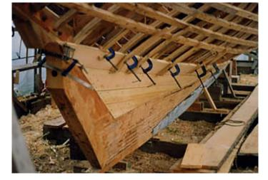
In my relative inexperience, I struggled with the first few strakes, trying each one four, five or six times, again thinking that this could take a lifetime. After a while, though, a rhythm developed, clamping became easier, and the work went along quite quickly.
