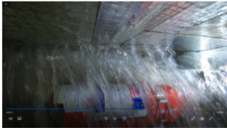
This image shows water inundating one of the hulls due to a deck gasket that does not seal properly.
